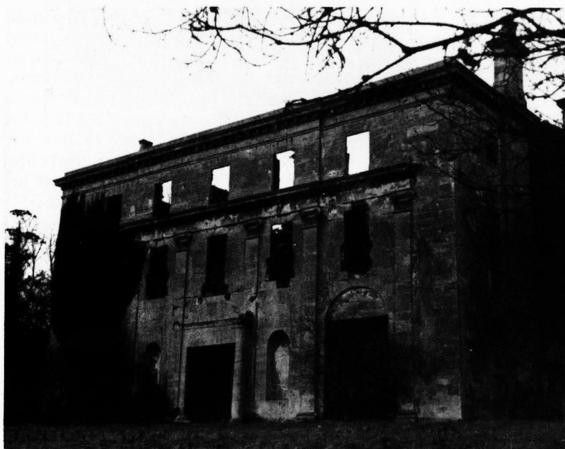
Piercefield House, St. Arvans, Gwent: the Soane Facade, showing shell damage.
