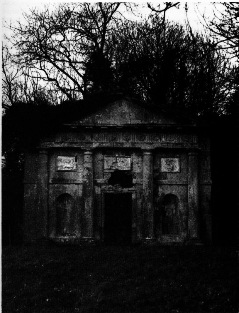
The East Pavilion at Piercefield House, also damaged by shells.
