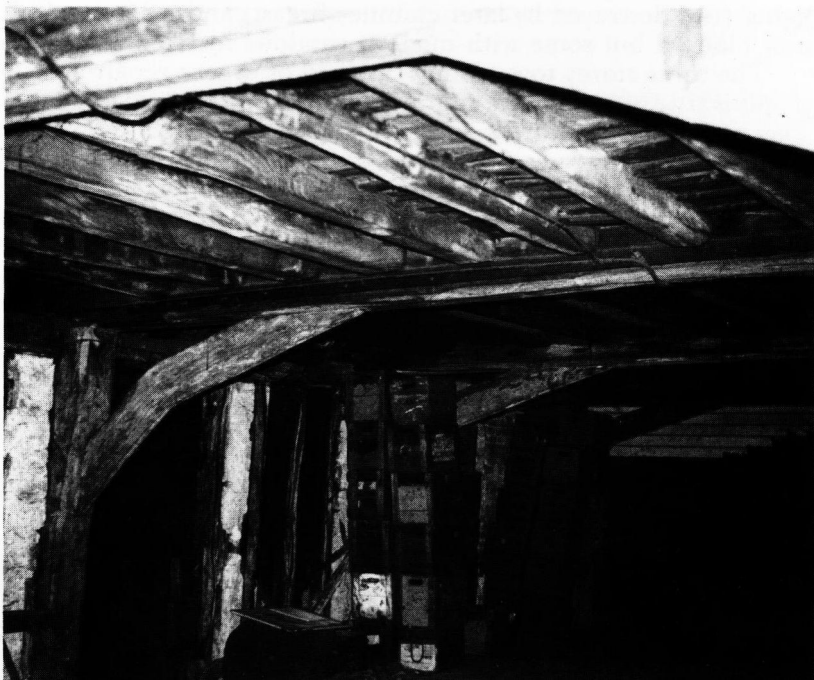
Early Tudor Warehouse, Ipswich, Suffolk, showing wall posts, tie beams and bracing on the first floor north-south range.
