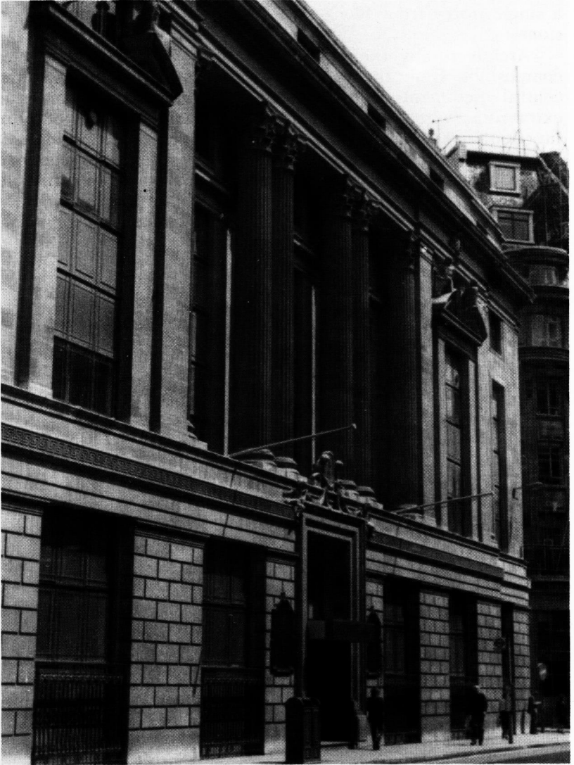
The former headquarters of the London Life Association, King William Street, City of London.
