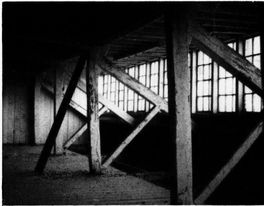
Framing on the top floor of the mill.
